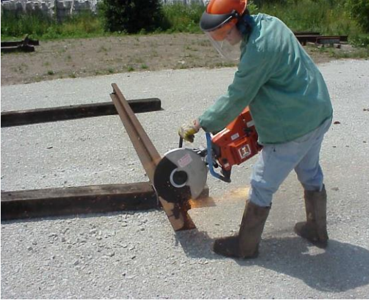
Top Rail Cutting
