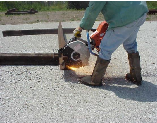
Rail Side Cutting View
